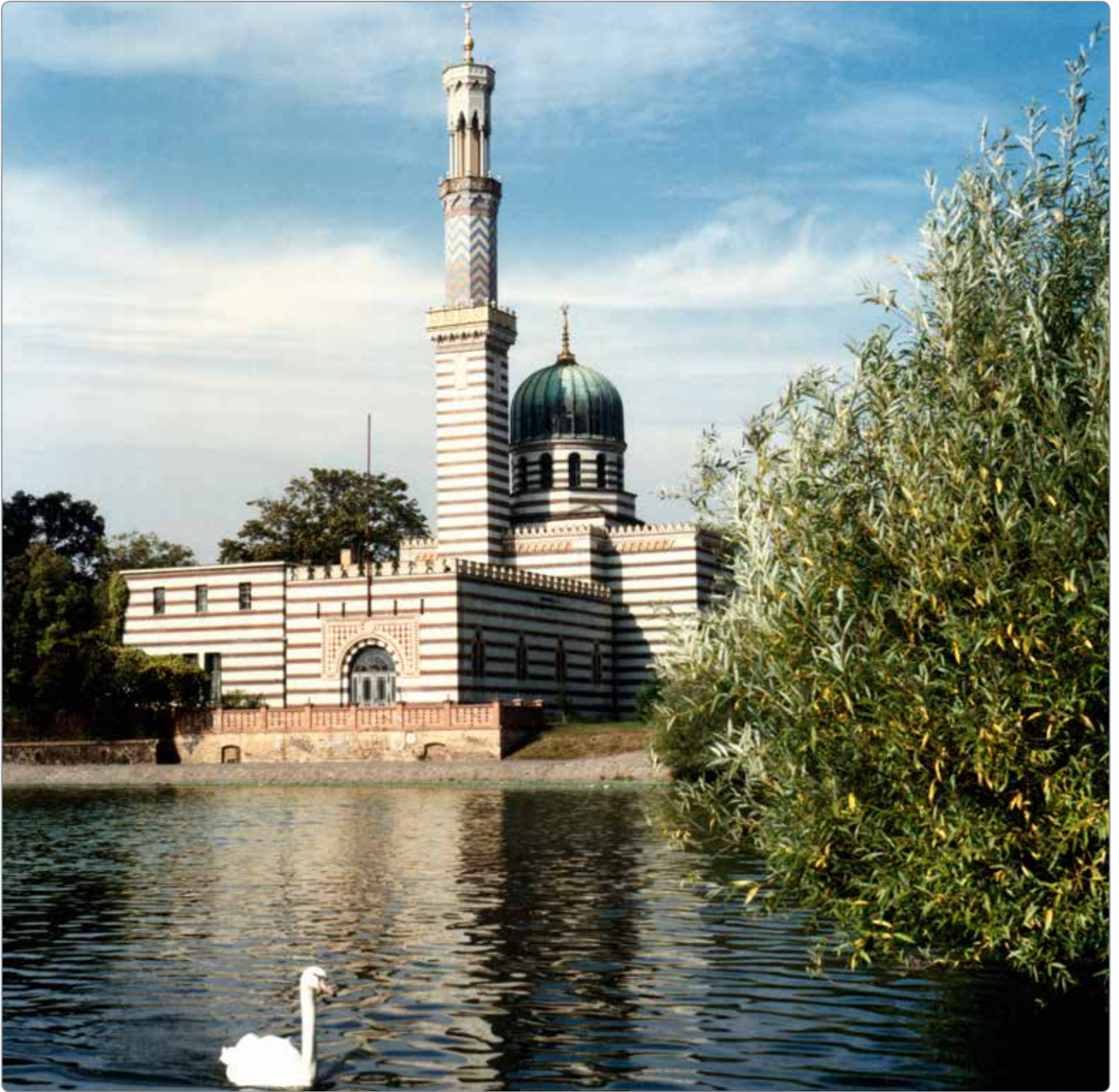
The pumping station for the Sanssouci Palace Gardens fountains, built in 1841-1843 in Islamic mosque architecture. (Photograph: Michiel 1972)
